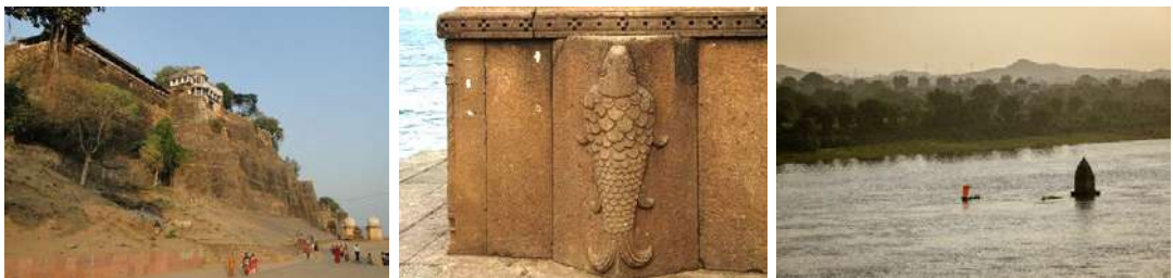
Figure 10: a) Outer wall of the fort b) Carvings related to natural elements of the river (fish in this case) on the platforms along the ghats to perform sacred rituals c) Temple submerged in the river at the time of floods (Location: Maheshwar, MP) (Source: Google Images)
